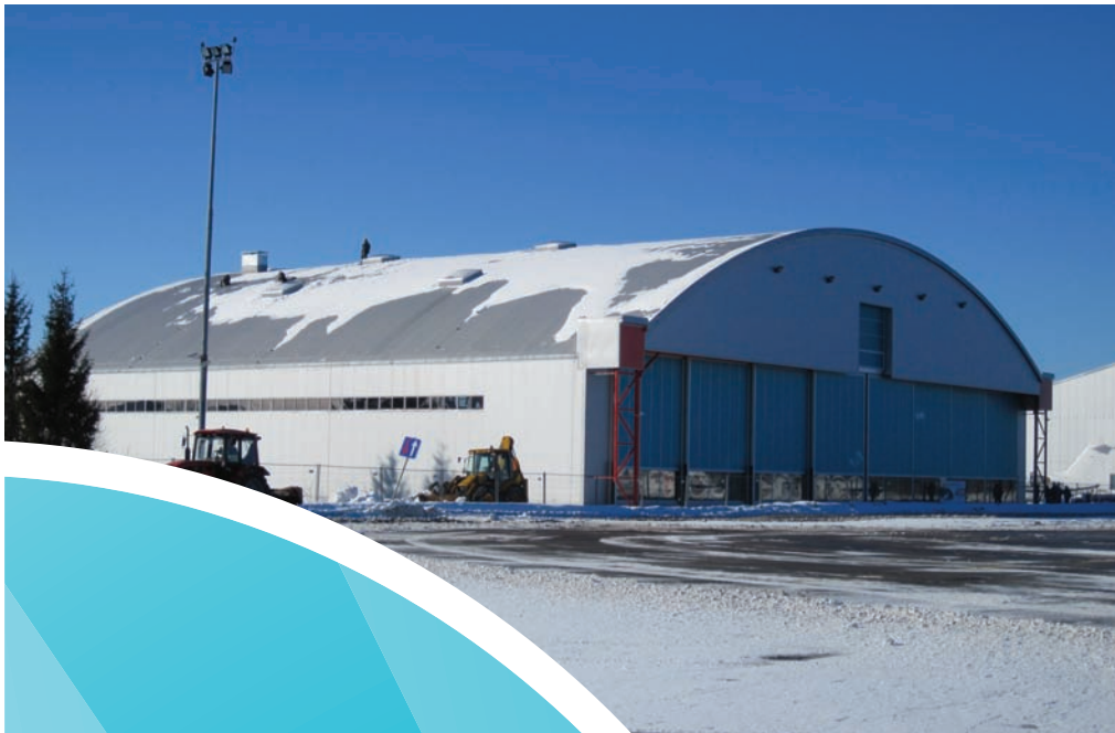
Above and right: BBAC's hangar at Riga International Airport
