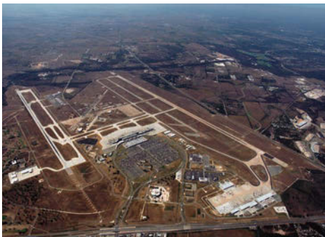
Above: Ascend has leased a 20-acre parcel of land at Austin Bergstrom International Airport
