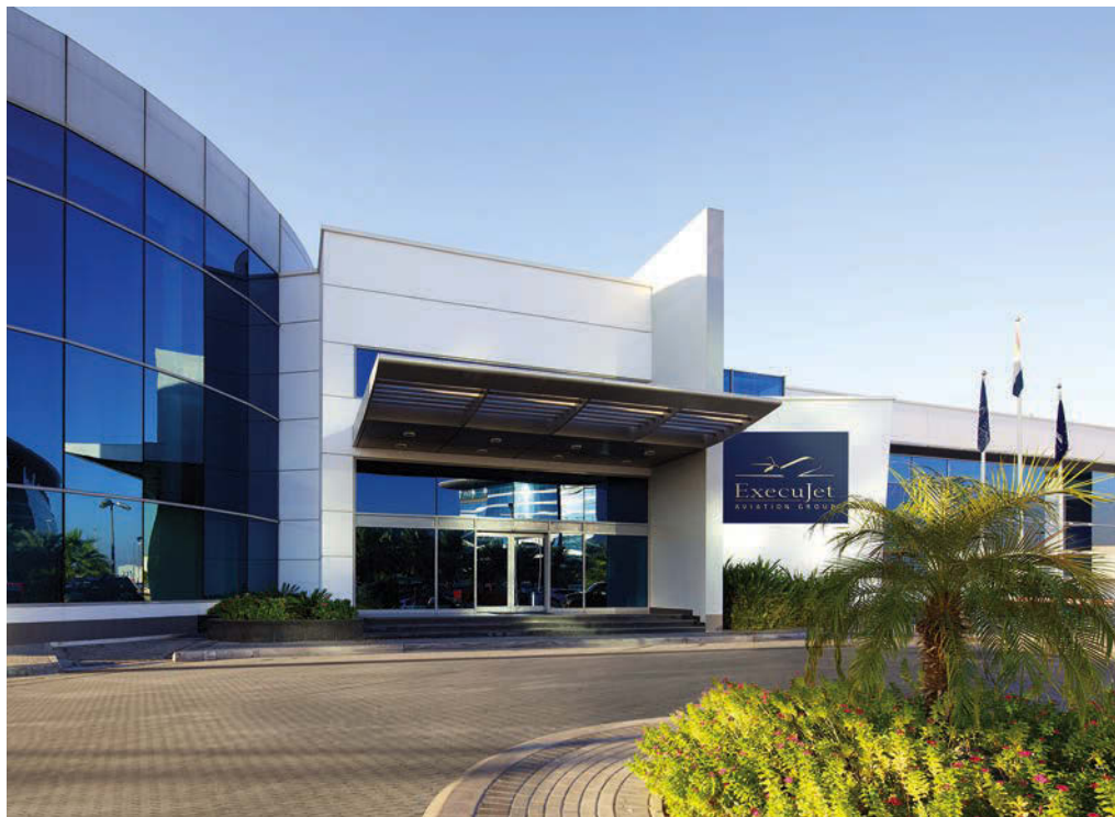
Above: ExecuJet’s FBO facility at Dubai International Airport
